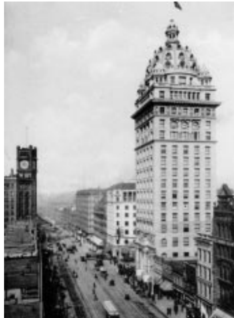
The Spreckels, or Call, Building, as it appeared after completion in 1898.
